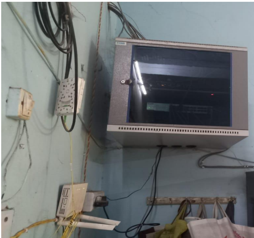
Wall mount Rack with Power Cable Manager in Staff Room
